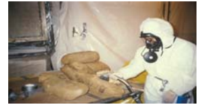
Objects were cleaned using a High Efficiency Particulate Air (HEPA) filtered vacuum and compressed air.
