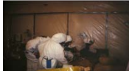
Smithsonian staff work with asbestos abatement contractors to handle and sort collections for cleaning.
