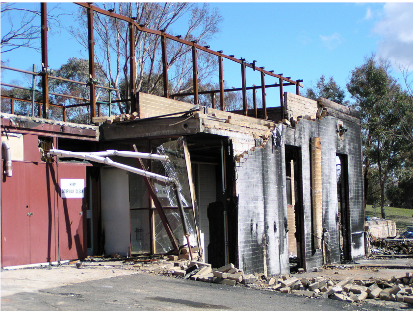
Top: A rear view of the main building before the fire. Middle and Bottom: Views of the building after the fire. The archaeological stores were located at the far end. The top photograph was taken from the Egan Insurance Report (2003).
