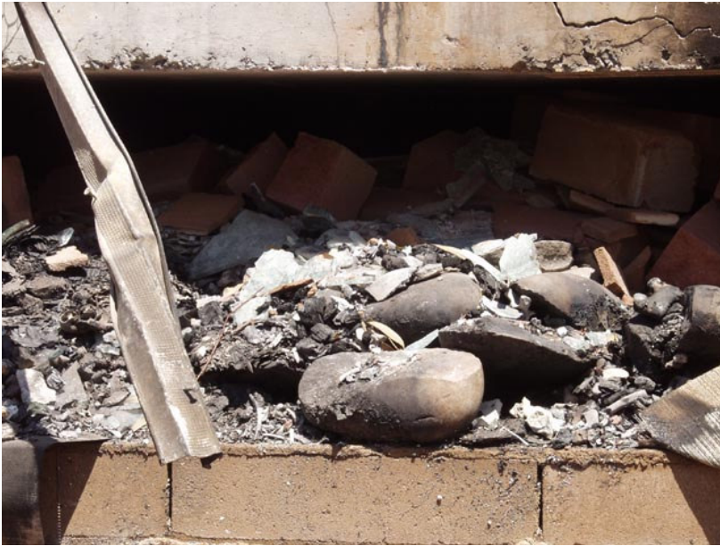
Artefacts and other retrievable remains could be seen wedged in between the upper and lower slabs where the storage room was previously been located.
